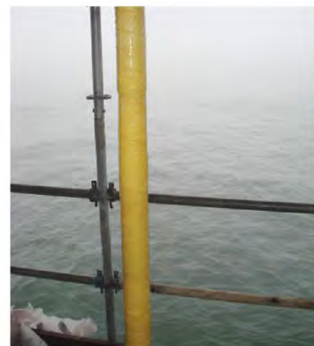
The pipe after it was repaired with STOP IT® HP™.
